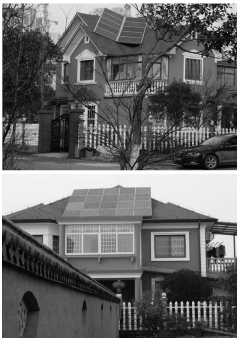
图1 江西省两处 5 kW 家庭太阳能光伏发电设施 Fig. 1 5 kW household photovoltaic systems in Jiangxi Province
